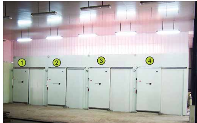
Photo 2 : A (4 day cycle) banana ripening room construction.
