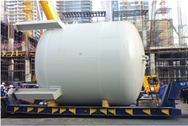
Photo 3: Expansion tank on ultra low bed trailer
