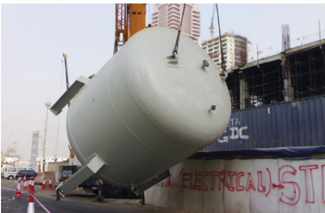
Photo 4: Expansion tank in the process of hoisting
