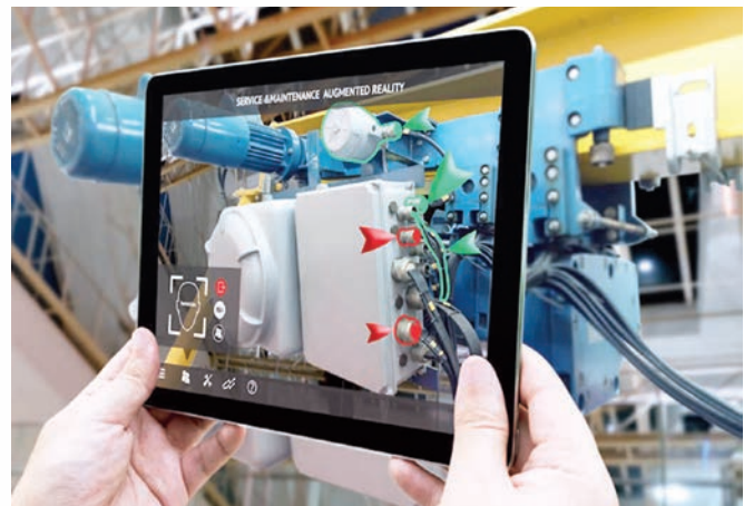
Figure 9: AR highlights the health of components with different colours, helping engineers to diagnose the problem
