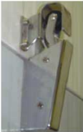
Hydraulic door closer ensures total closure of the cold room door, thereby avoiding cold air from escaping, and saving energy.
