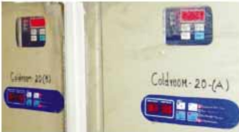
Microprocessor controller provides smooth and continuous operation by timer-activated defrost cycles.
