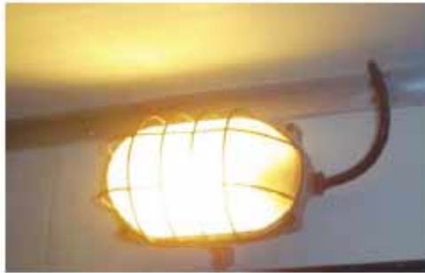
Vapour proof interior light to illuminate the cold room.
