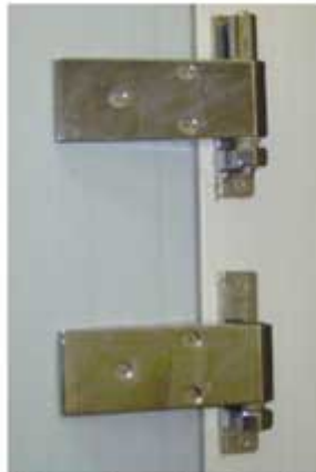
Spring action self closing door hinges serve as an important feature in preventing the door from remaining open.
