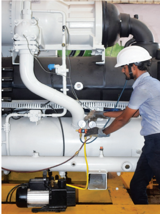
Figure 2: Technician fixing manifold to chiller
