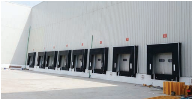
Distribution centre with insulated panel construction and docking facilities
