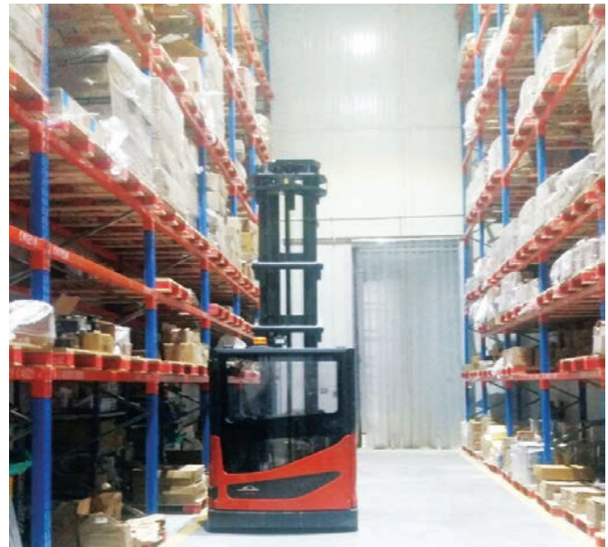
Palletized storage inside cold chamber with material handling equipment
