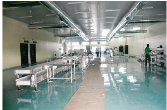
Process hall in a pack house
