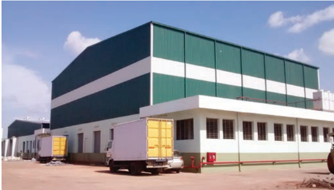
A multi-facility project with pack house, ripening chamber and commercial multi-product cold storage at Kappec, Hubli
