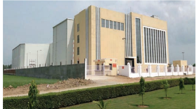
Palletized convertible multipurpose cold storage project (8000 pallets) with fully automated PLC based control system at Boxco Logistics, Sonapat Haryana
