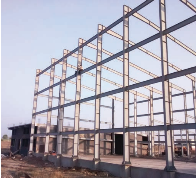
A PEB structure
