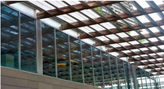
Photo 2: Perforated metal louvers
