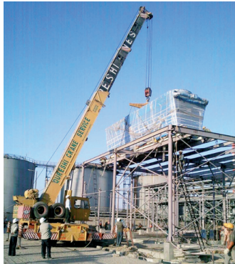
Figure 3: Adiabatic cooler being installed at Hindustan Zinc, Udaipur
