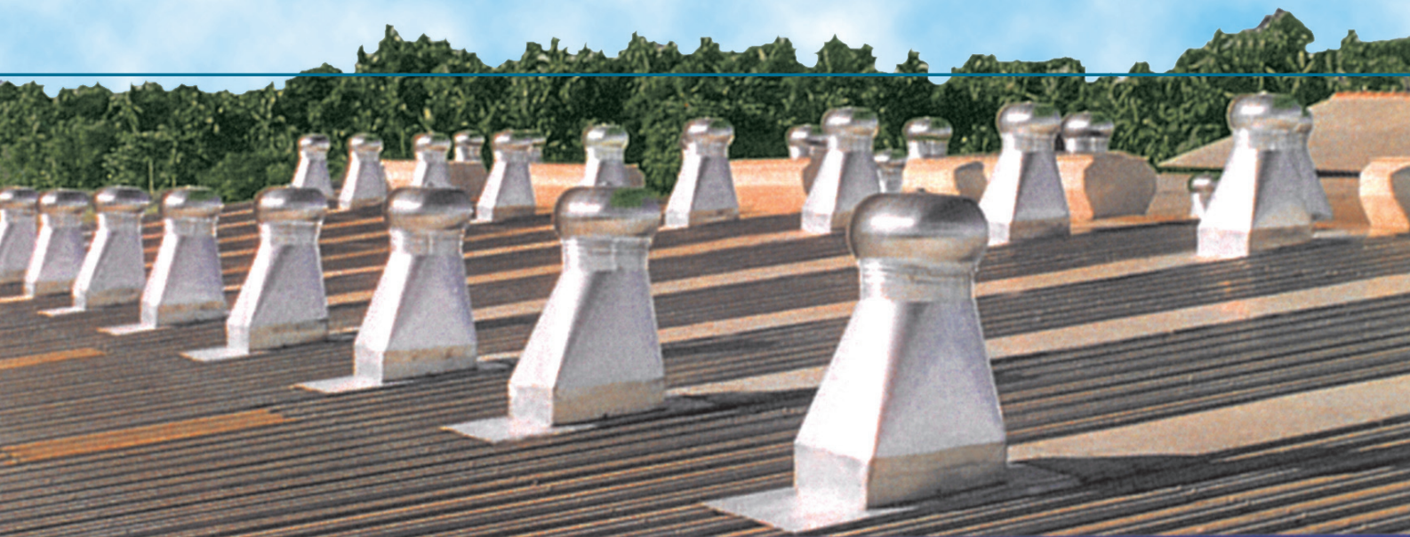
Turbine ventilators installed on the roof of a factory for natural exhaust.
