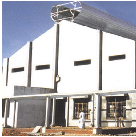
Figure 2 : Natural gravity roof-ventilator.
