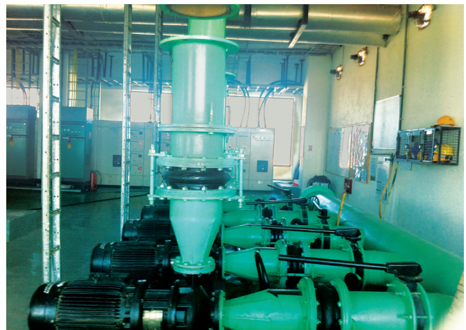
Figure 6: In-line pumps – after retrofit
