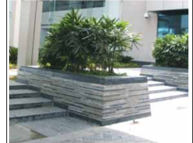
Stone waste as finishing material for planters
