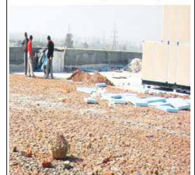
Broken bricks reused for brickbat coba
