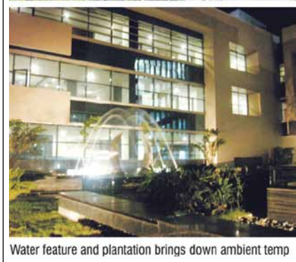
Water feature and plantation brings down ambient temp The courtyard at Patni Campus
