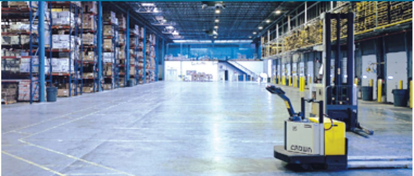
Interior of a modern refrigerated warehouse with a 40 ft. to 60 ft. wide area for staging or arranging in the proper place.
