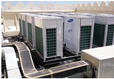
Photo 3: VRF outdoor units installed on the terrace with architectural camouflage.
