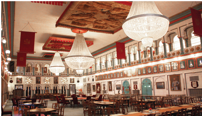
Photo 1: Durbar Hall with new AHUs installed.
