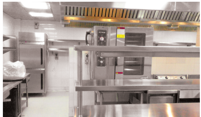
Photo 4: A view of the new kitchen for the banquet hall.
