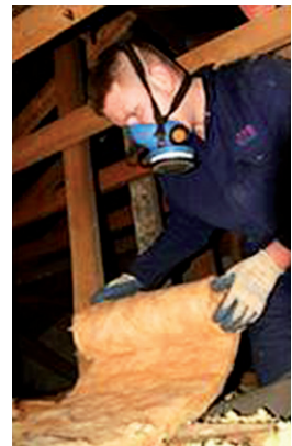
Figure 12: Safety gear is required for application of open cell insulation
