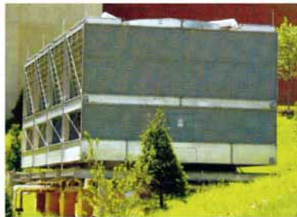
Hybrid wet-dry closed-circuit cooling towers.
