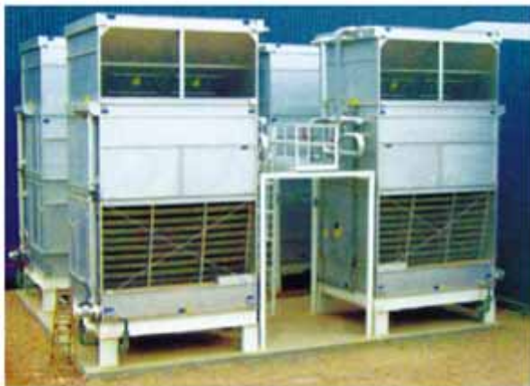
Crossflow cooling tower installation on sports arena.
