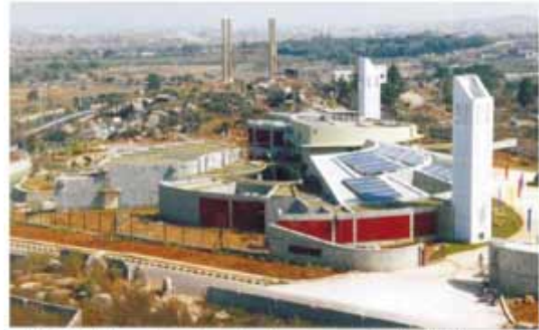
GBC building showing wind towers and solar PV system.
