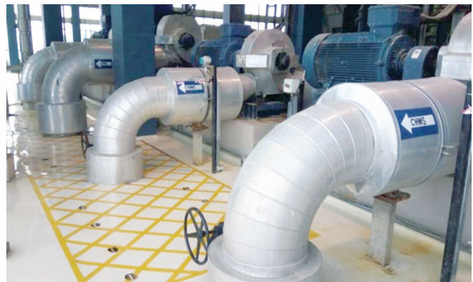
Figure 9: Chilled water pipe routed below the ground trench
