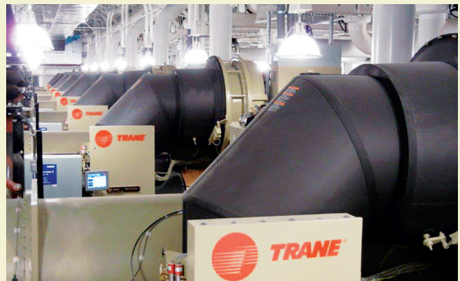
Trane CenTraVac multi-stage centrifugal chillers at a job site in Masdar City, UAE
