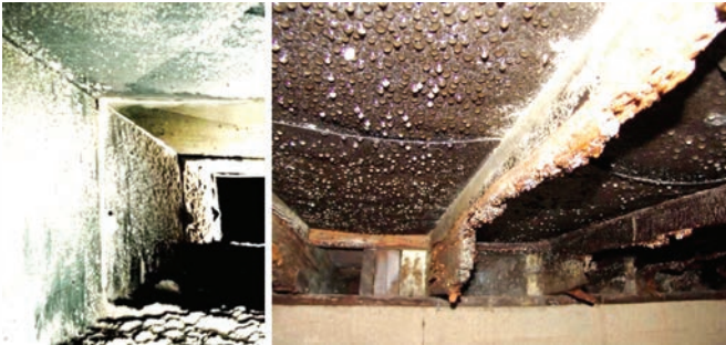
Figure 2: Duct contamination
