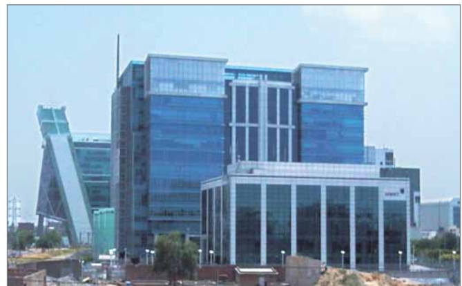
Photo 2: A commercial building of one million sq. ft. functioning with an Energy Centre
