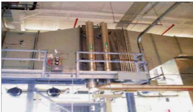
Figure 8: Inlet air cooling of gas turbine
