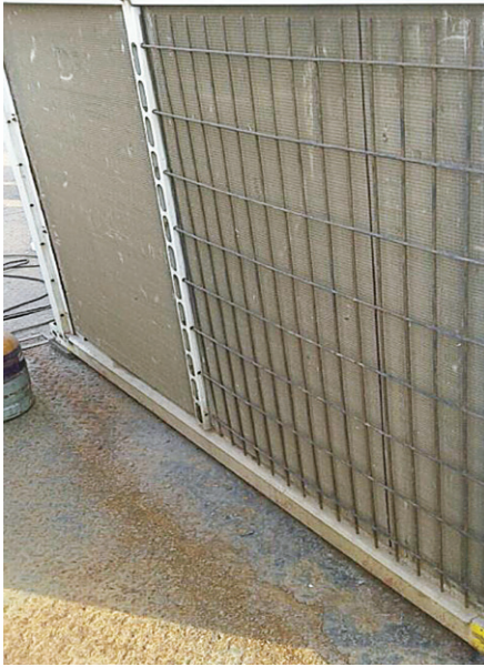
Photo 1: A dirty coil before the coating process
