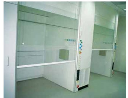
Photo 6 : Walk-in fume hood.
