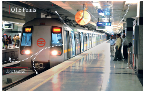
Figure 16: Platform level air distribution
