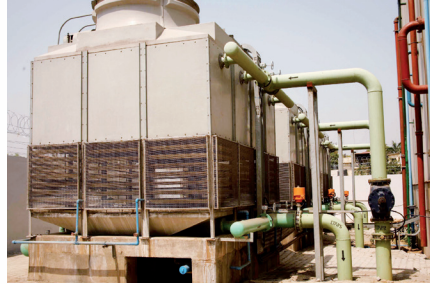
Figure 14 : Cooling tower installation
