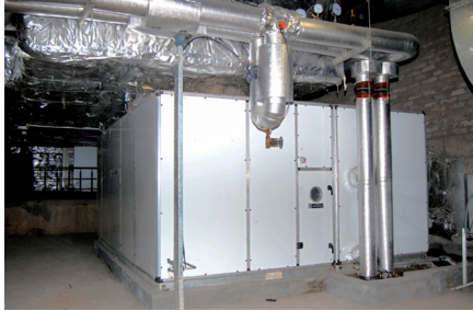
Figure 13 : AHU installation
