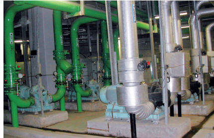
Figure 12 : Pump installation
