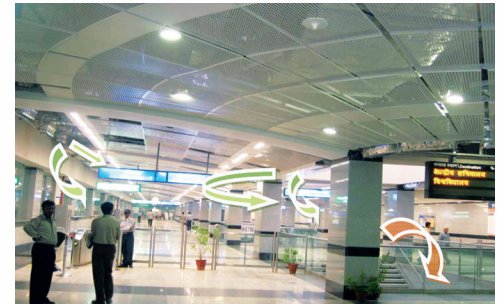
Figure 17: Concourse level air distribution
