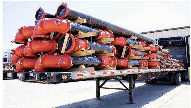
Grooved prefabrication minimizes transportation costs and site impact
