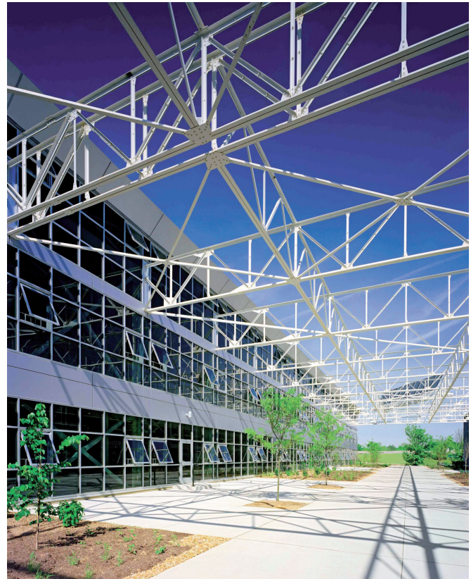
The LEED Platinum rated Alberici Headquarters in the United States uses grooved mechanical pipe joining
