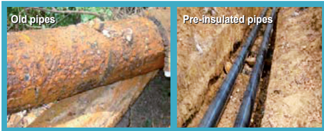
Figure 2: Damaged old pipes replaced with pre-insulated pipes
