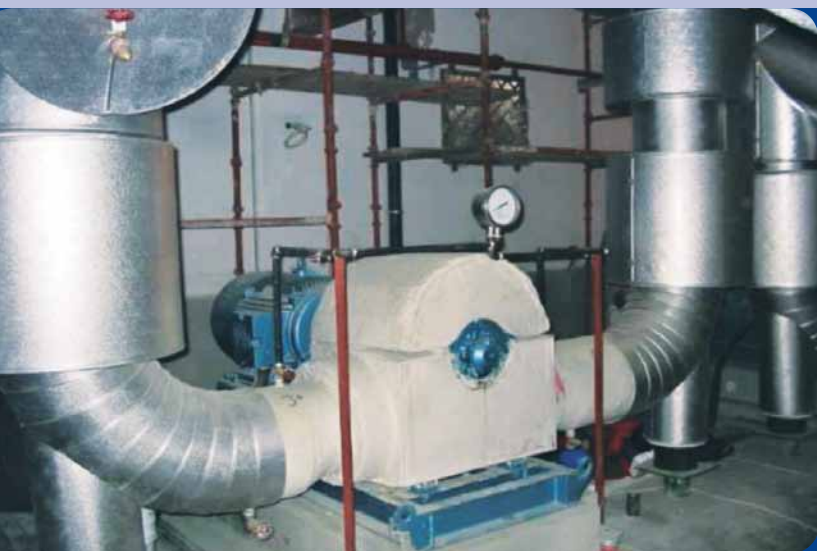
Stucco aluminium cladding gives a good finish to insulation
