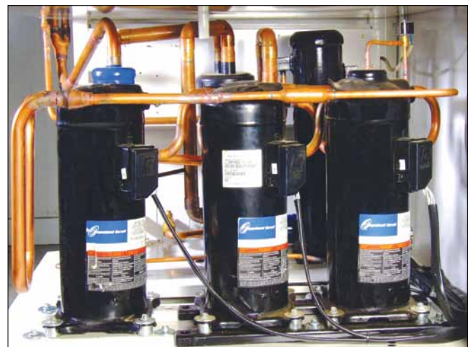
Chart 6 : Mechanical architecture with Digital Scroll.
