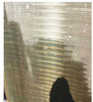
Figure 14: Restored coil after fin cleaning and nano coating
