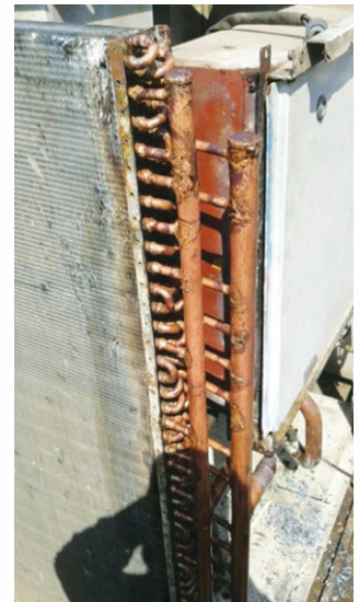
Figure 12: Chemically cleaned and coated header
