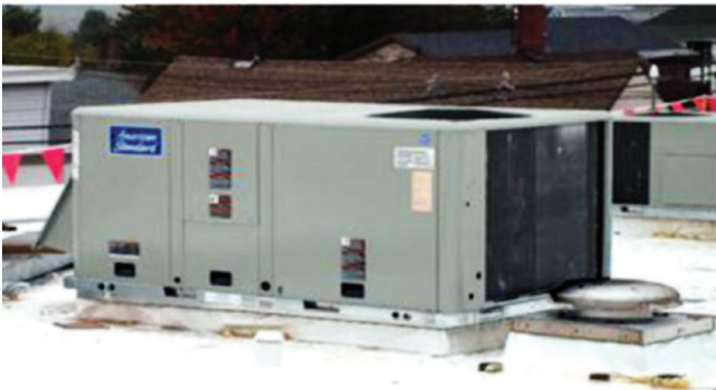
Photo 7 and 8: Roof top units using low charge ammonia systems at Roche headquarters in the U.K.
