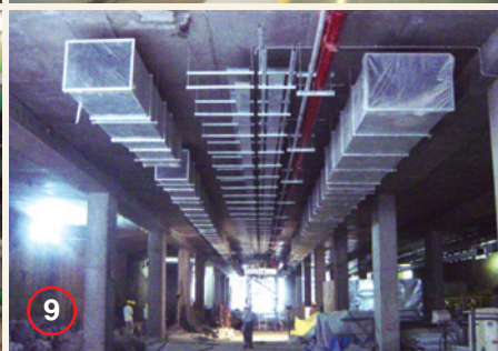
1 An underground tunnel during construction. 2 Construction activity at Connaught Place, in the heart of the city 3 A completed tunnel 4 Stairs connecting platform to Concourse 5 The Concourse level of a typical station 6 A train arriving at a platform 7 Passengers entering the train while others are on their way out 8 Chiller plant room at ground level 9 Air distribution ductwork for the cool supply air 10 When the job is over and garlands handed out, you must have a photo for memory's sake.
