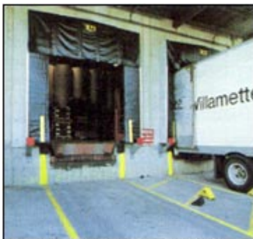
Loading bay seals or dock shelters create a barrier that helps to keep warm air and humidity from entering the cold store area.
