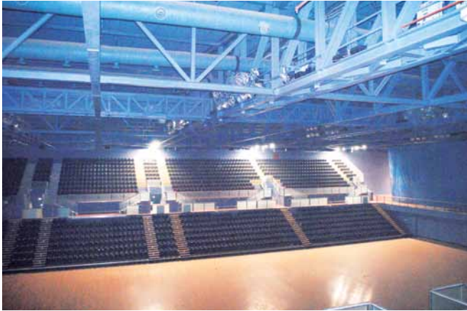
Inside view of the badminton court with exposed ductwork
