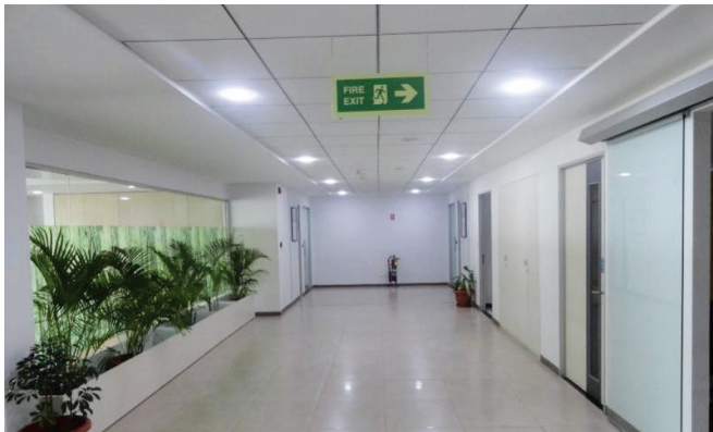
Figure 2: Efficient LED lighting in the building
