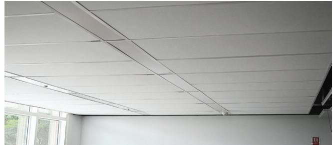
Figure 3: Uponor radiant panel system
