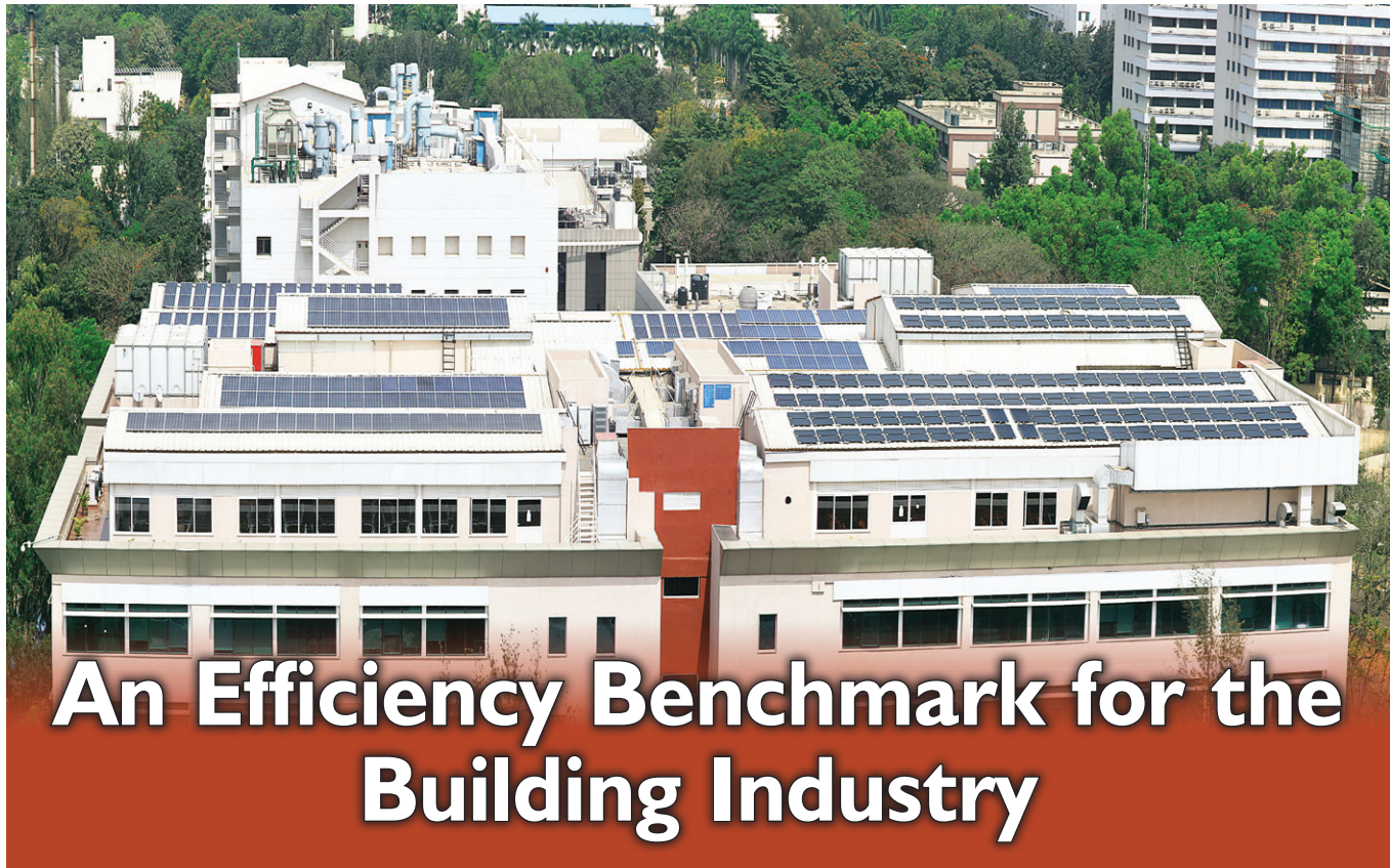
A panorama of solar PV systems on the roof of Infosys EC-53 building
