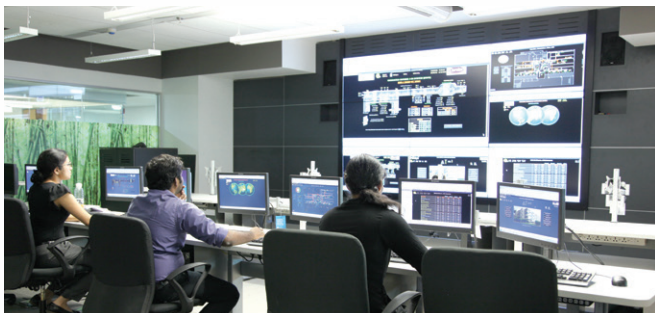
Figure 5: Central Command Center for monitoring performance
