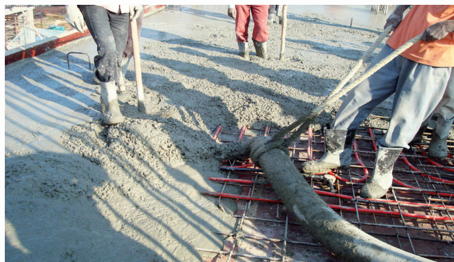
Figure 3: Concreting of slab with radiant pipes
