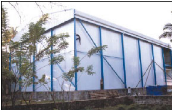
Photo 2 : The 'Dutch Barn' construction design of cold store for Snowman Frozen Foods, Kochi. Photo courtesy of Beardsell Ltd.
