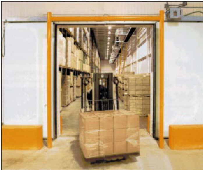
Photo 6 : A typical protection barrier in the shape of a goalpost with a Bi-Parting Horizontal Sliding Power Operated door. Courtesy of Jamison Door Co., USA
