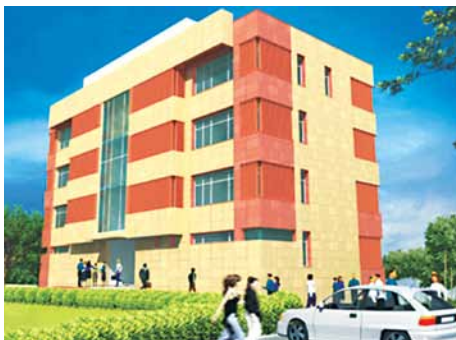
Photo 2 : North West view.
