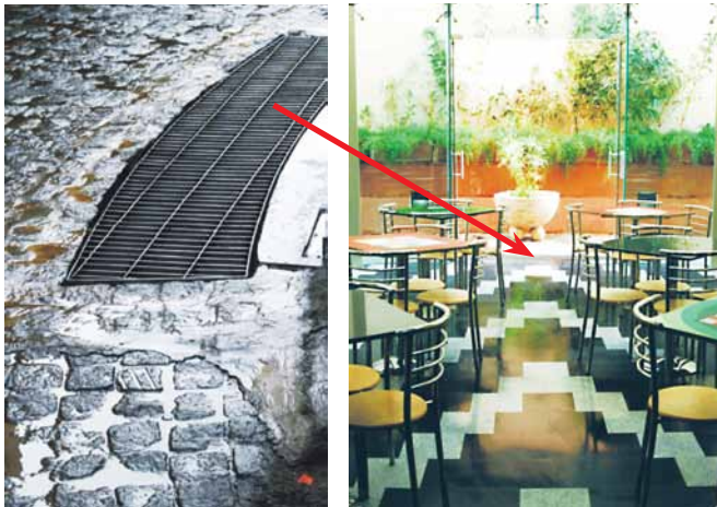
Photo 9 & 10 : Gratings at the entrance of the staff canteen.
