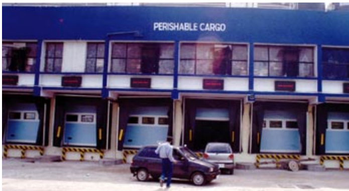
A row of Dock Shelters, Sectional Overhead Doors and Bumpers for speedy unloading of cargo from trucks at the Truck Dock
