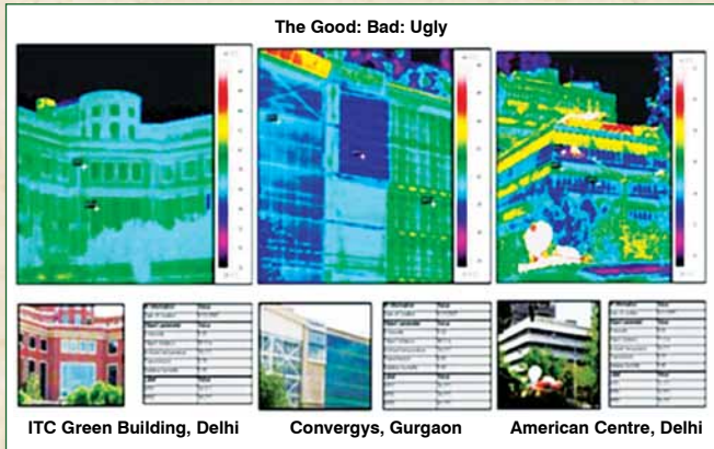
Photo 1 : Thermographs of three different buildings, showing the leakage of cold air in blue. Note the building on the extreme left shows virtually no leakage (Source: www.greenpeace.org/ India/ press release)
