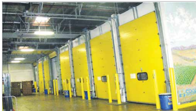
Photo 3 : Outside view of the ripening rooms
