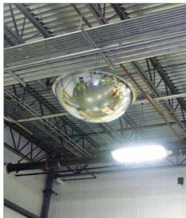
Photo 16 : Hemispherical mirror for safety of operators
