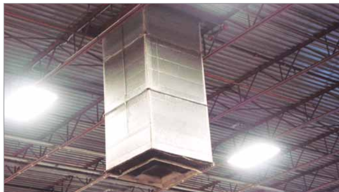
Photo 10 : Duct piece for evaporative cooling air inlet
