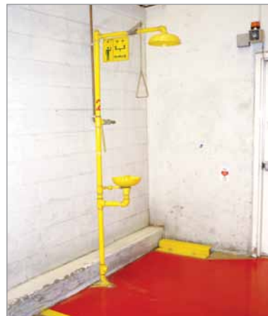
Photo 17 : Water shower and washing area for emergency treatment
