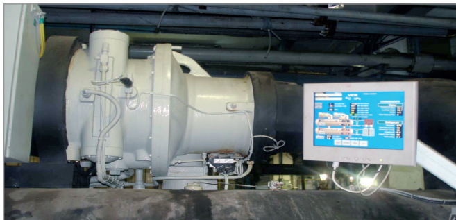
Figure 11: Energy efficient centrifugal chiller
