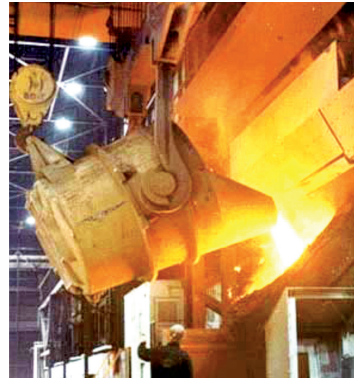
Figure 7: Existing practice of steel making is a cause of fugitive emission
