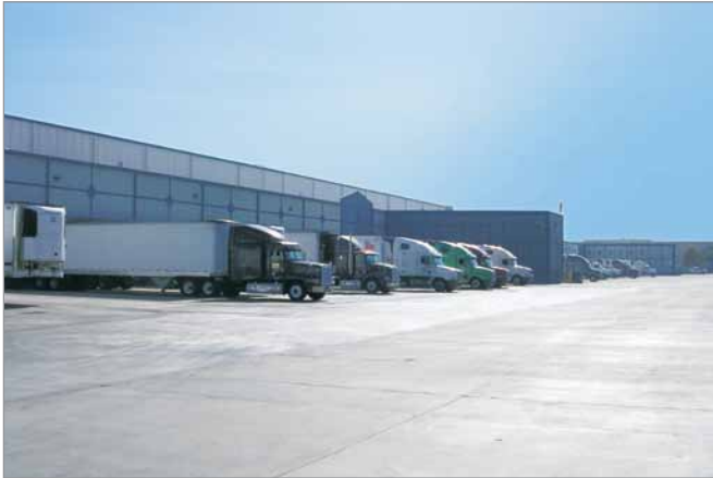
Photo 18 : Containers docked at a DC
