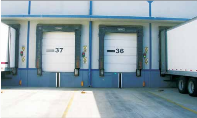
Photo 25: Dock doors from the outside
