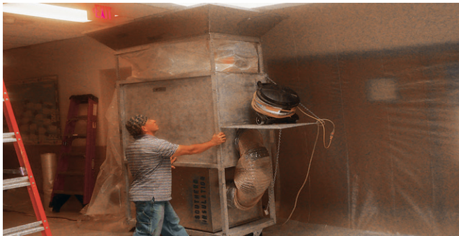
Photo 8: Insulation removal using portable hood.
