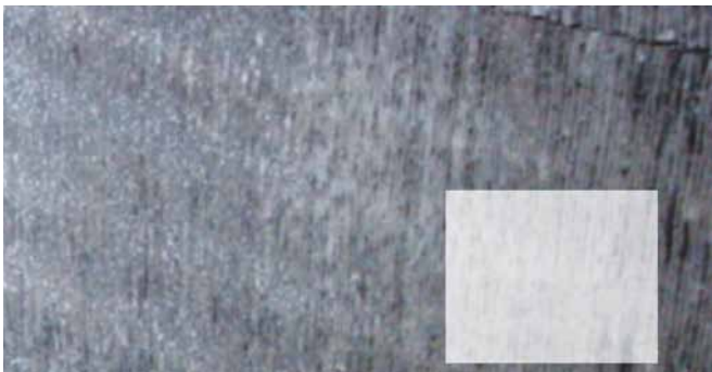
Figure 4: View of the AHU cooling coil after cleaning.
