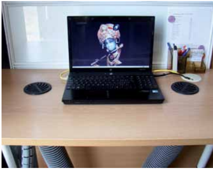
Figure 6: Task or Desk cooling terminal
