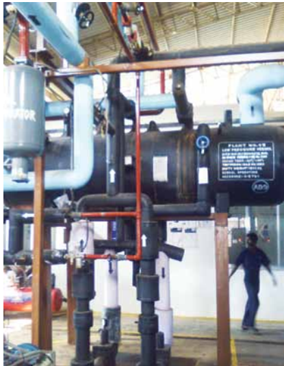
Figure 8 : Low pressure vessel in operation
