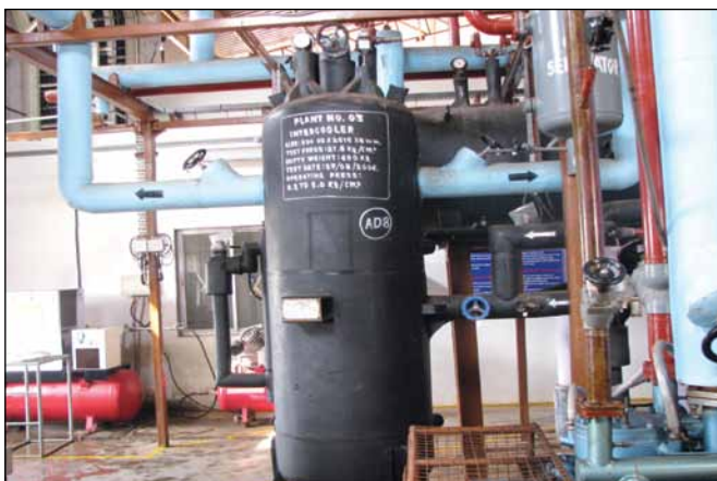
Figure 5 : Open flash cooler.
