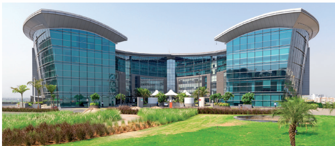
Figure 4: Software Park at EON Special Economic Zone, Kharadi, Pune
