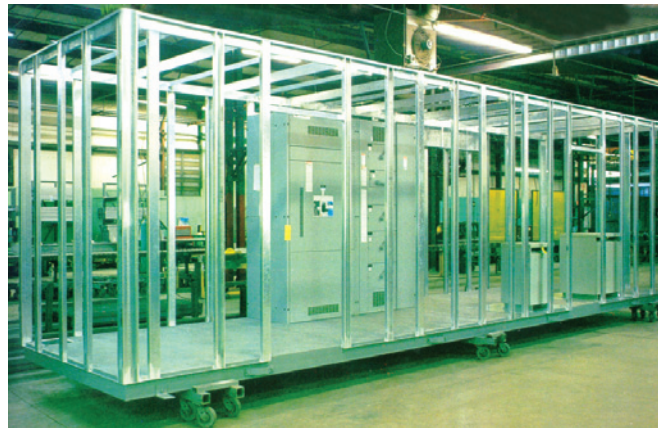
Photo 2 : Steel channel base and galvanized steel rolled sections form the structural skeleton for a prefabricated machine house.
