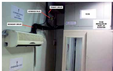
Figure 3: Test rig of PLTSS with water as PCM
