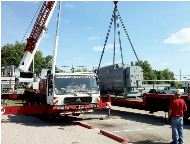
Figure 7: Adsorption chiller being loaded on a trailer
